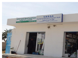
Commercial shop of the water user association
